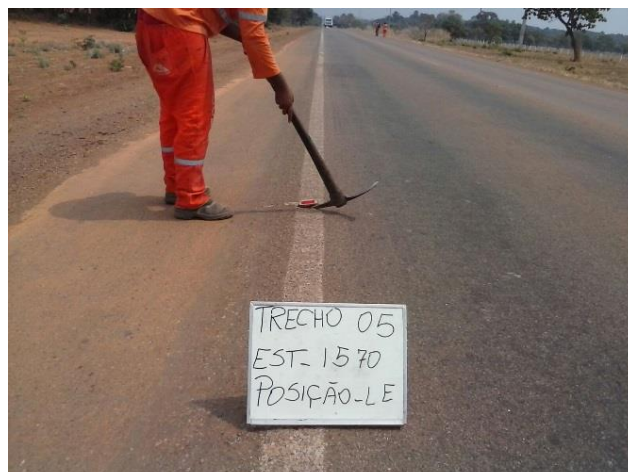
Figura 34 – Removendo as tachas refletivas
