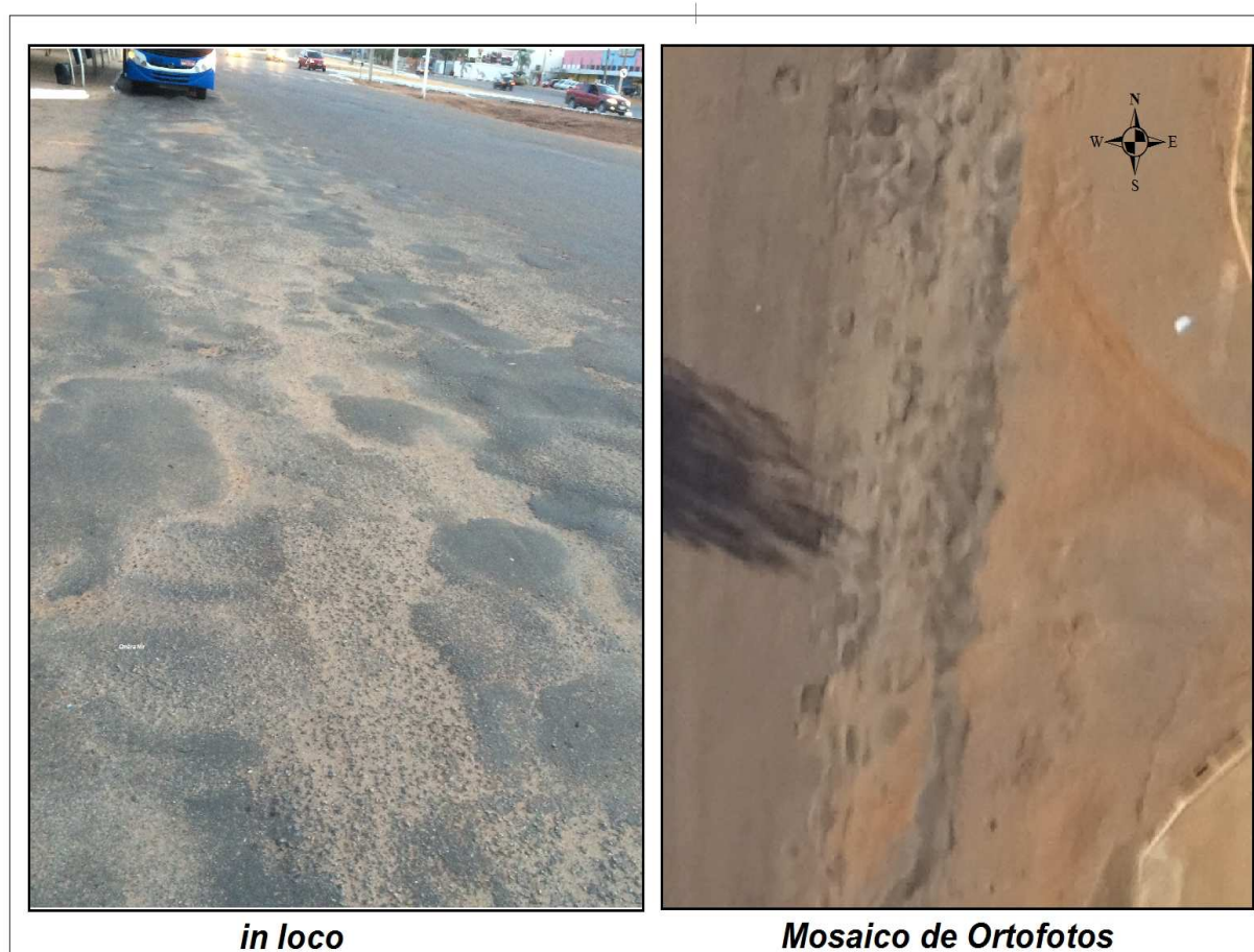
Figura 16 – Remendo emergencial
