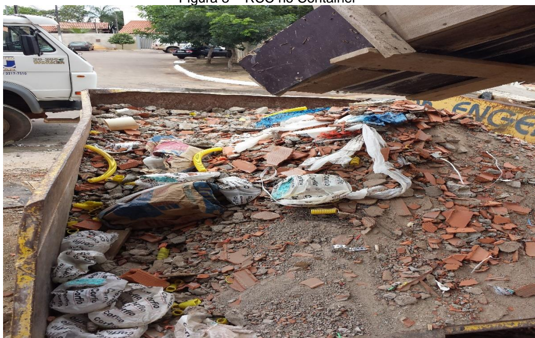
Figura 3 - RCC no Container
