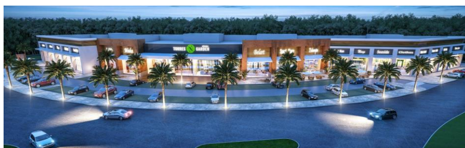
Figura 8 – Fachada Principal Torres Garden
